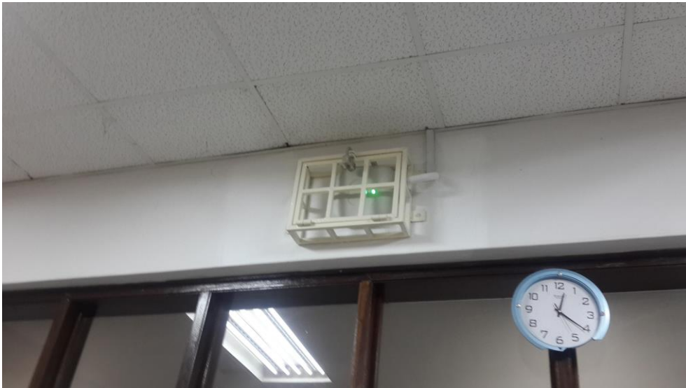
Figure 2: Physical security of access points
