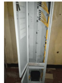
Indoor ODF Installation
