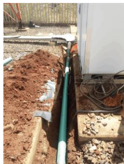
Site Entry Installation
