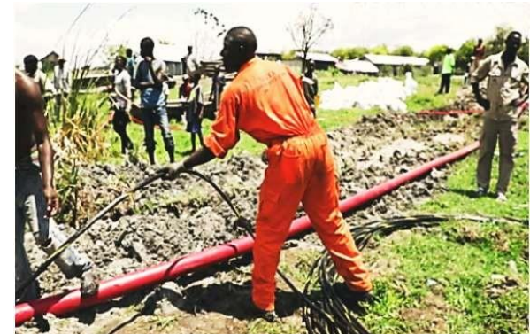
Submarine cable being pulled to the shore
