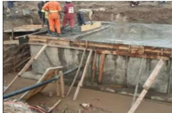
Beach manhole construction
