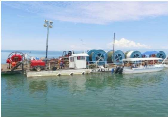
A fully prepared cable laying barge
