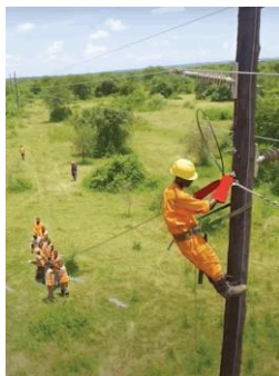
Overhead Fiber Stringing
