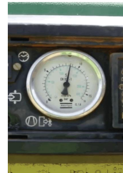
Duct Integrity Test
