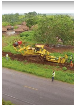
Duct Installation
