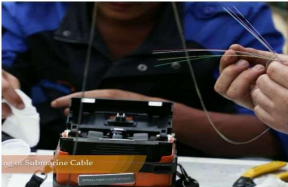
A submarine joint being spliced
