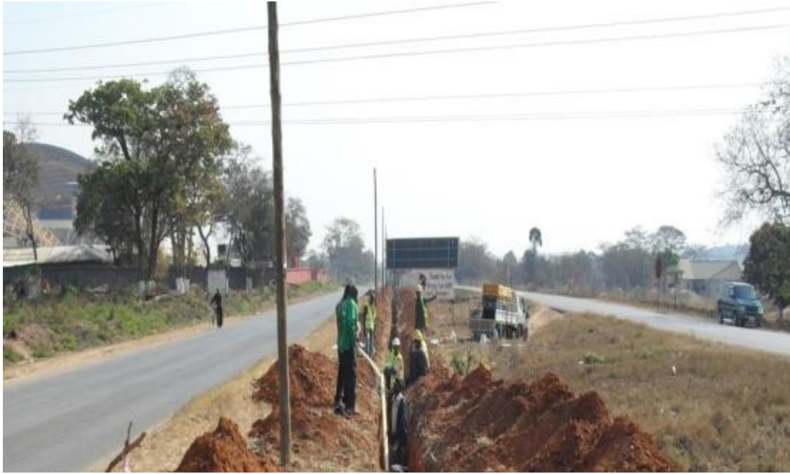
Figure 4: Construction works on Direct Optical Fiber in Ndola.
