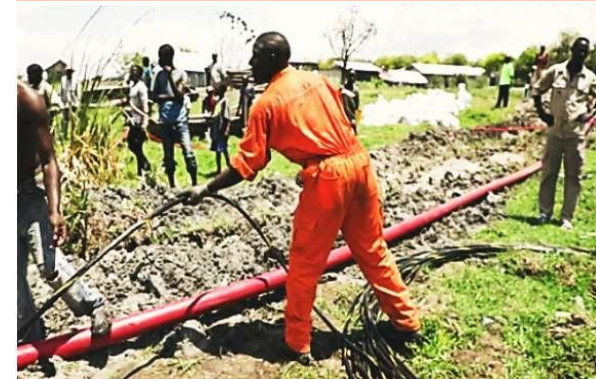
Submarine cable being pulled to the shore
