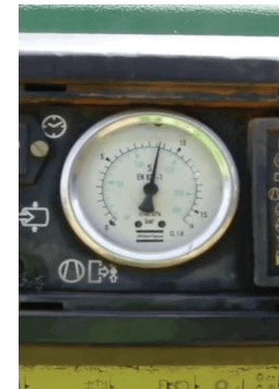
Duct Integrity Test
