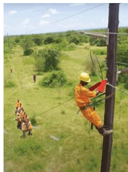
Overhead Fiber Stringing
