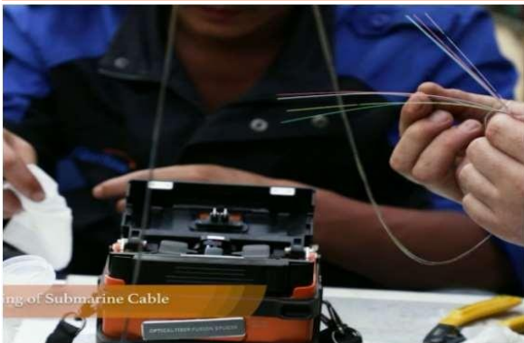
A submarine joint being spliced
