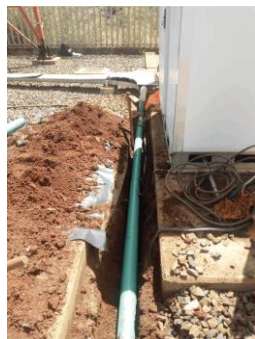
Site Entry Installation
