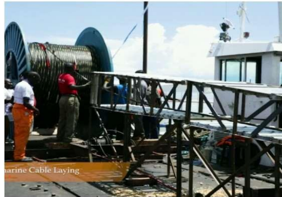
Submarine cable being laid in water
