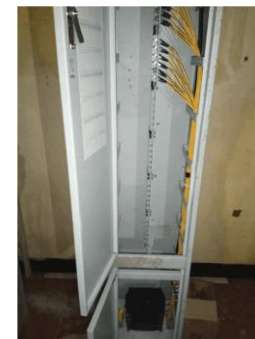
Indoor ODF Installation
