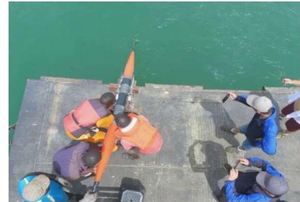
A fully assembled marine joint being laid in the water
