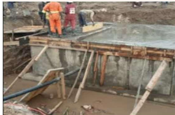
Beach manhole construction
